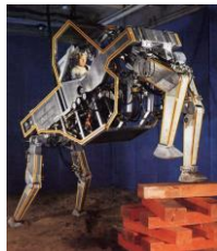
Figure 1.52: R. Moshier at General Electric(1968): quadrupled walking machine (11 ft tall, 3000lb)
